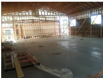
Good progress being made on the hall.
