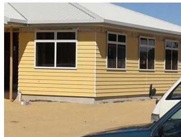
The windows are now in the offices.
