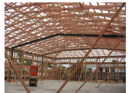
Figure 3 The view inside the new hall
