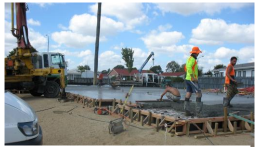
Figure 1 Pouring the concrete foundation
