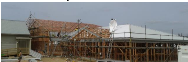
Figure 4 The roof goes on the new building
