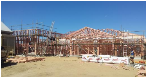
Figure 2 The framing goes up for the new centre
