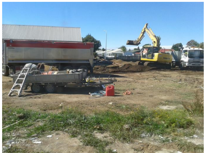
Excavating the site
