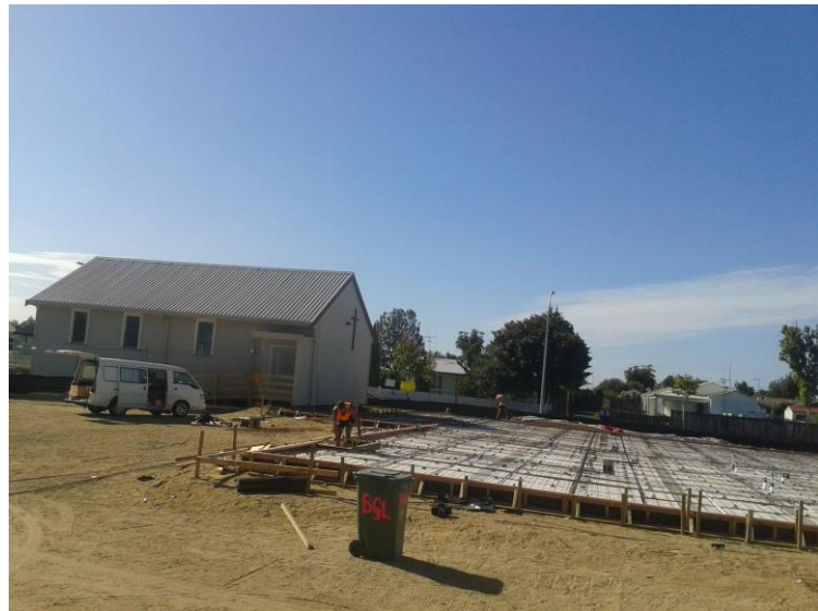
Ground prepared and ready for concrete to be poured
